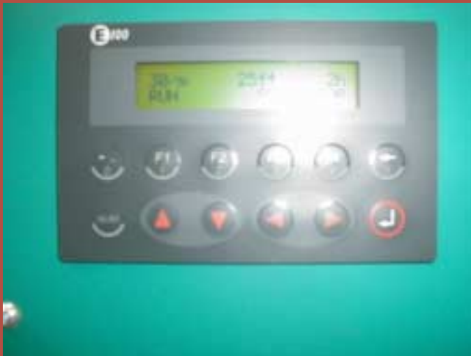
HMI read out from sensor
